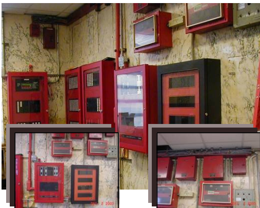
Below: Fire Alarm Improvements
