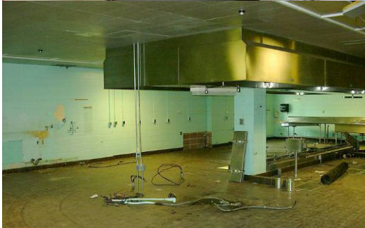
Top: Major plumbing, electrical, and HVAC upgrades
