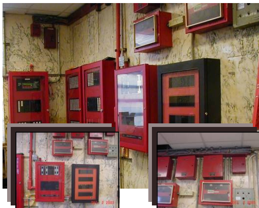
Below: Fire Alarm Improvements
