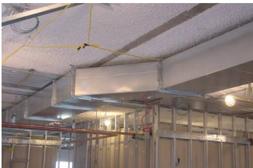
Below: HVAC renovations meet new load requirements
